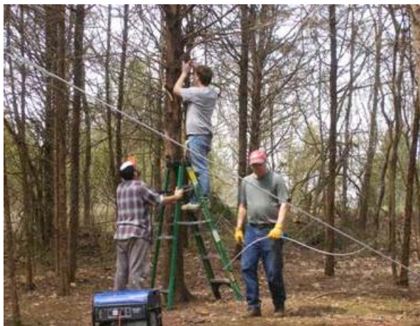
Installing steel cables for the traverse at the ropes course
